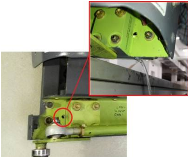
Clean Drain Holes in Window Frame Assembly:
