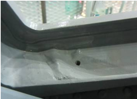
Clean Drain Holes in Window Sill (Structure):
